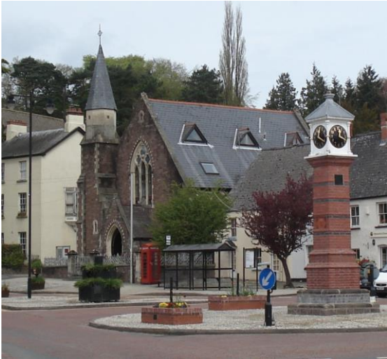
Fig.44 The former Congregational Church, Twyn Square, one of the few buildings in this part of the conservation area to use unpainted stone
