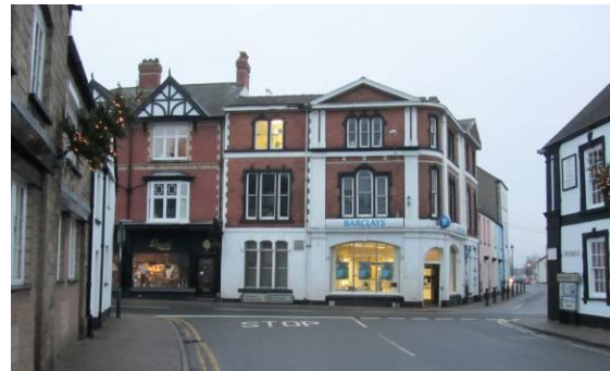
Fig.137 Barclays Bank, from Porthycarne Street
