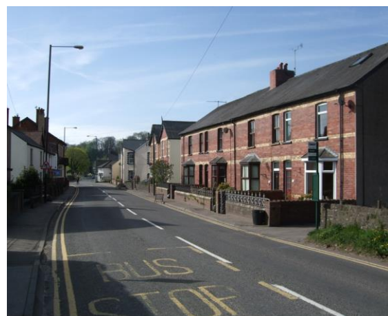
Fig.85 A view looking south into the conservation area along the A472. Note the well-defined townscape which forms the approach to the conservation area which includes a good survival of cast iron railings
