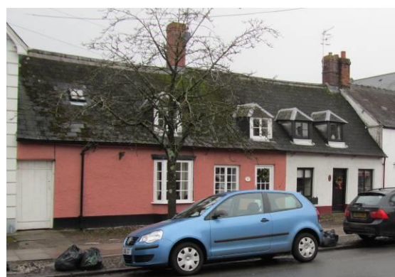
Fig.115 The Woodcutters Cottage, Maryport Street.
