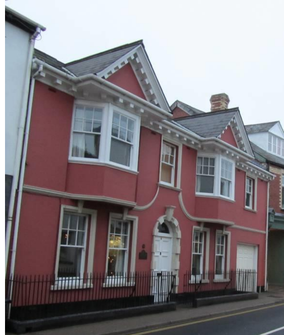
Fig.151 Portland House, No.4 Bridge Street. Queen Anne style Edwardian building.
