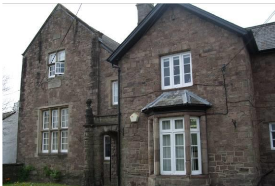
Fig.159 Former school with squared stone and ashlar
