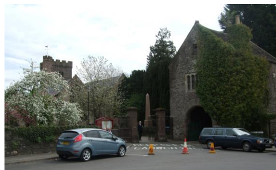
Fig.66 The church of St Mary and the Priory Gatehouse form an important group to the corner of Church Street and Priory Street
