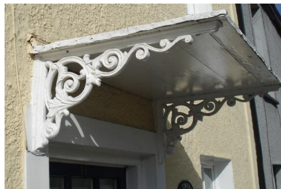
Fig.37 Cast iron decorative brackets to door hoods – a distinctive pattern which is repeated on a number of notable buildings
