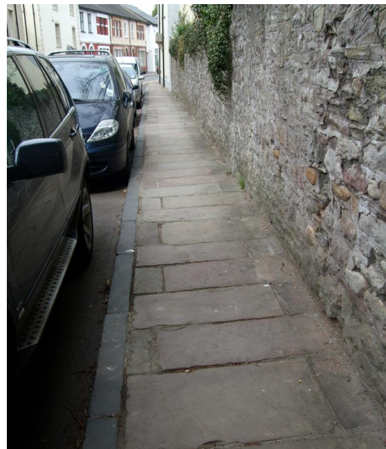
Fig.73 Section of historic stone boundary wall to the north-east side of Priory Street. The combination of stone boundary wall and traditional paving make up part of the general high quality of the public realm to this part of the conservation area
