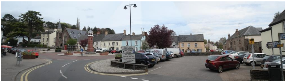
Fig.43 The north-east side of Twyn Square – a subtle but attractive variation to the roofline culminating in the gable and stair turret of the former Congregational Chapel adds considerable character to the townscape of this part of the conservation area
