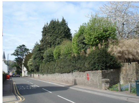
Fig.59 The long stretch of rubble stone boundary wall to the north-west side of Castle Parade is Grade II listed and forms an important historic element giving structure and definition to the street scene
