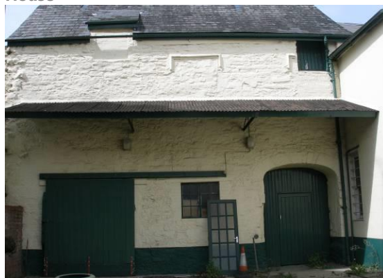
Fig.106 No.28 Bridge Street.
