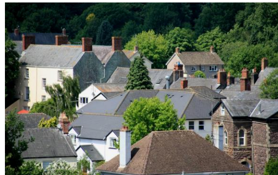
Fig.163 The varied roofscape of the town, natural slate dominates
