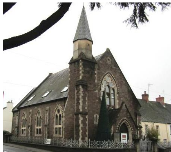
Fig.142 The former Congregational Church.
