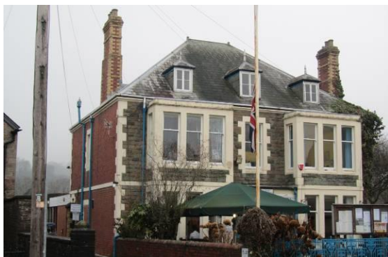
Fig.148 The Conservative Club, a well proportioned Victorian House
