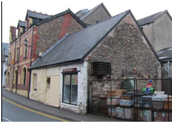
Fig.109 Former outhouse behind the former Cardiff Arms on New Market Street.
