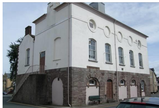
Fig.132 The Town Hall, south and west elevations. The ground floor arcading was infilled in the later 19 th century.
