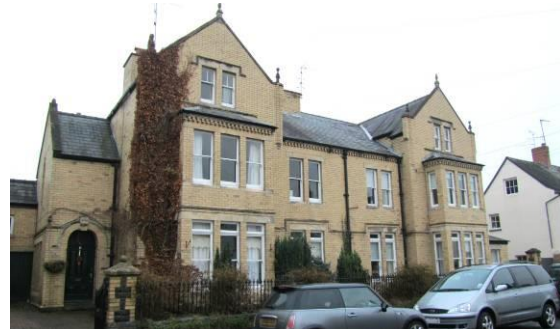
Fig.146 Double Villas in Victorian Jacobean Style, New Market Street
