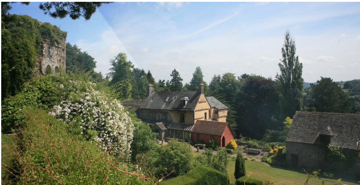
Fig.61 The Gatehouse, its outbuildings, Castle House, the barn and sections of the inner ward form the best surviving group of elements of Usk Castle. They can only really be appreciated from inside the castle
