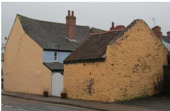
Fig.111 Storehouse to rear of the Old Bakery
