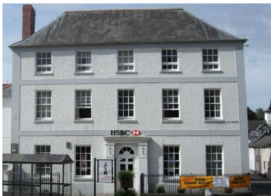
Fig.122 HSBC Bank Twyn Square, a prominent former Georgian townhouse.
