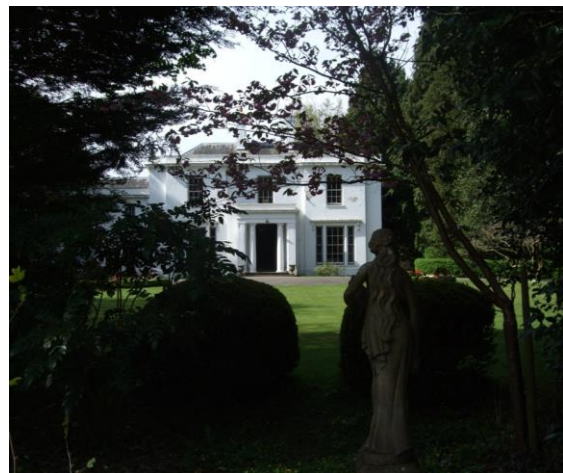
Fig.52 Porthycarne House seen through its landscape screen from the roadside
