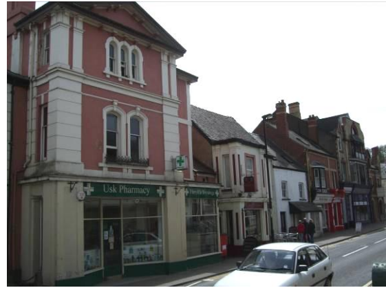
Fig.136 The Usk Pharmacy, Bridge Street
