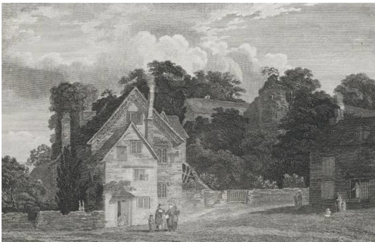
Fig.8 Mulberry House, Twyn Square with the castle ruins behind, 1801
