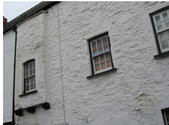
Fig.102 Part of the Great House of Roger Williams, in Old Market Street, illustrating some of the subtlety of the construction, which raises questions regarding the age of its construction.
