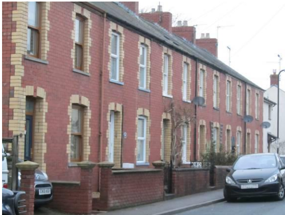
Fig.117 Late 19 th century red brick terrace in Mill Street.
