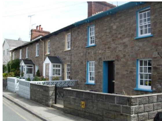
Fig.33 A terrace of more modest cottage-style houses to Baron Street (Grade II listed) contrasting with the grander houses forming a group with the Town Hall
