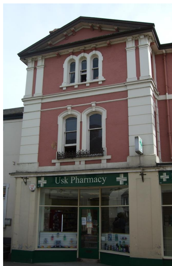
Fig.19 Windows, door architraves and quoins are painted to accentuate these architectural details emphasizing buildings with this treatment in the street scene – pictured No. 59 Bridge Street
