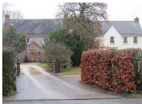
Fig.155 Recent houses, south side of Four Ash Street.
