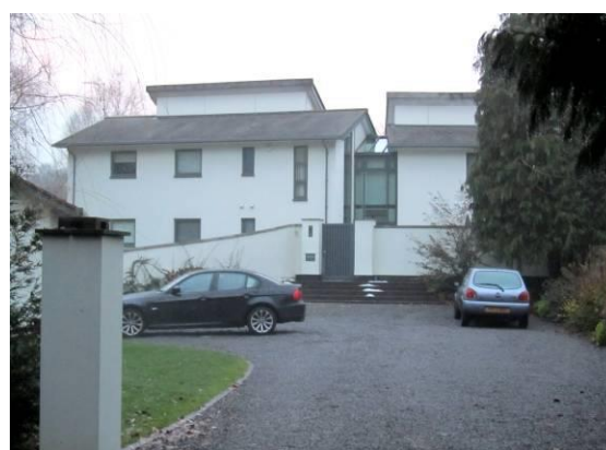
Fig.156 Recent houses at Porthycarne Gate.
