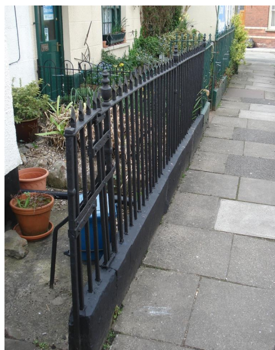
Fig.38 A typical set of cast iron railings to small front gardens, these examples may date to the late 18 th century
