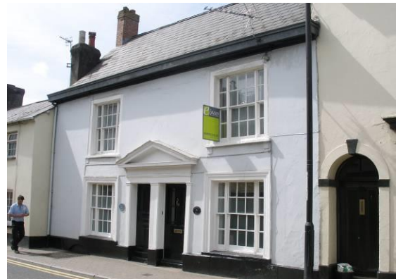
Fig.127 Gordon House, Bridge Street
